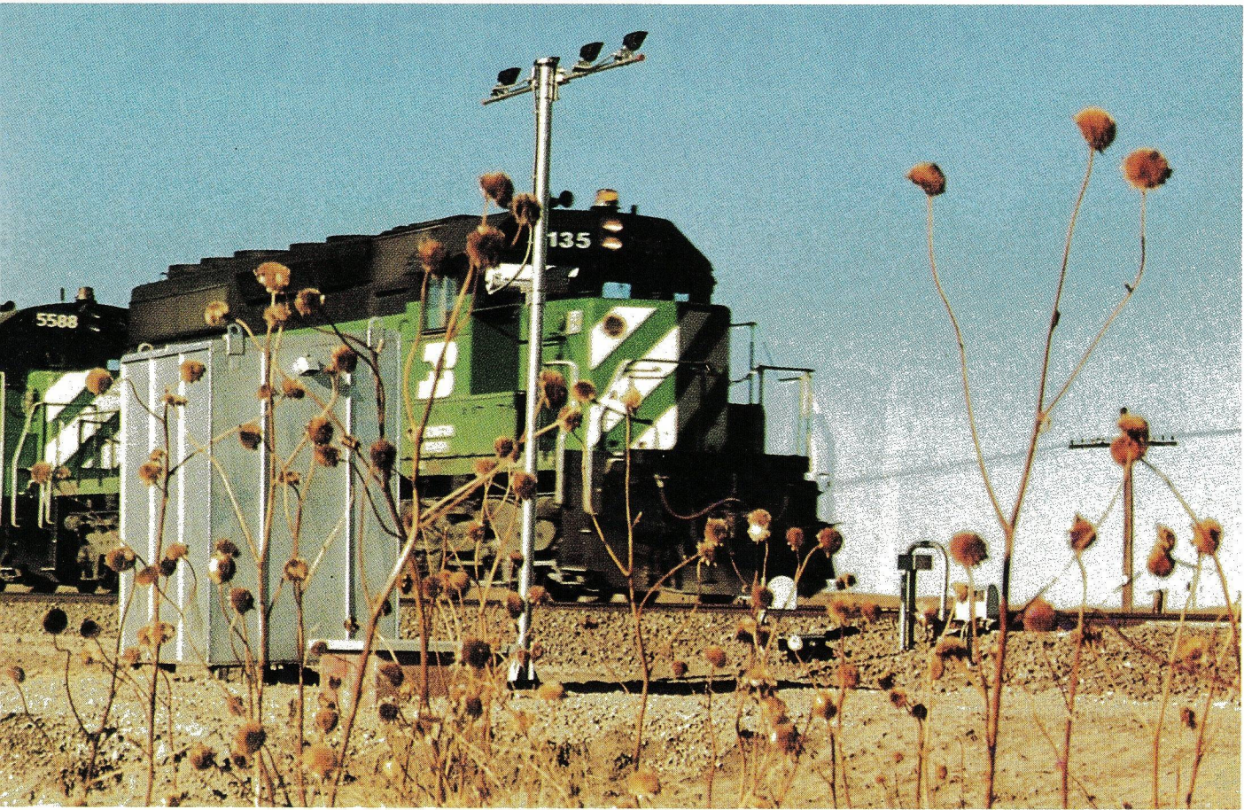
BN/Servo acoustic hot-bearing-detection systems are now installed at six locations. Fine-tuning continues.
